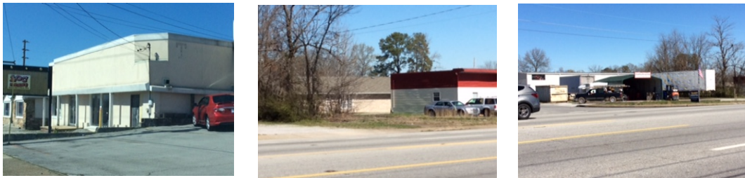
Evidence of abandoned & vacant properties on Ringgold Road and poorly maintained properties
